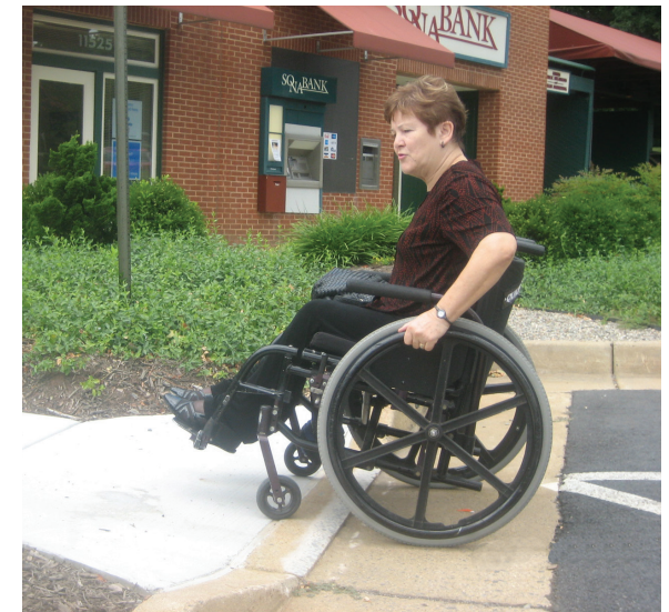
Curb ramp improvements made by Tetra Partnerships, Inc., at the Sunrise Valley Center, June, 2008.
